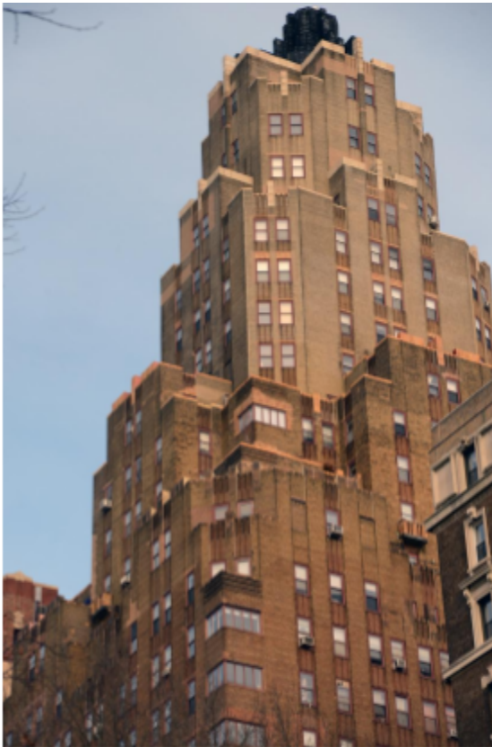
The Master Building, Riverside Drive at 103rd Street
